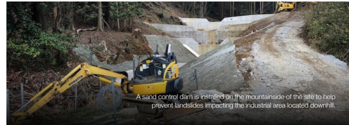
A sand control dam is installed on the mountainside of the site to help prevent landslides impacting the industrial area located downhill.
